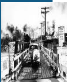
Stoney Creek Bridge November 19, 1946
